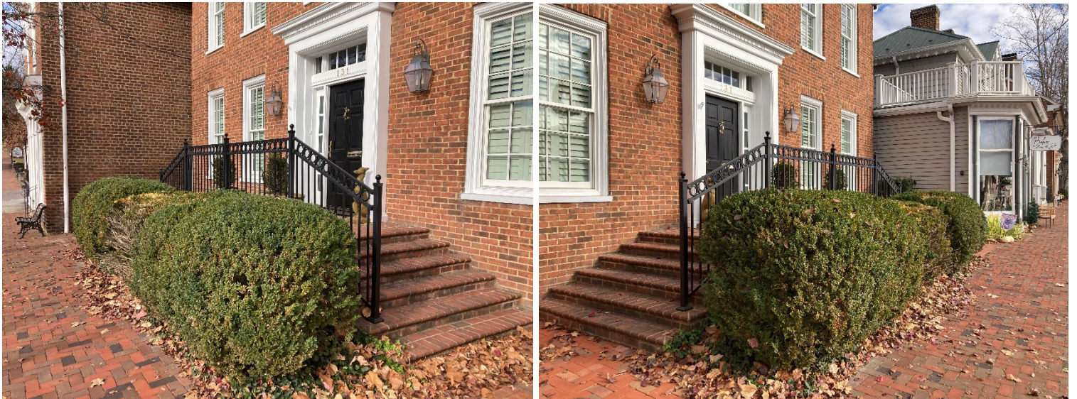
View of unapproved metal railing as seen from E. Main Street
