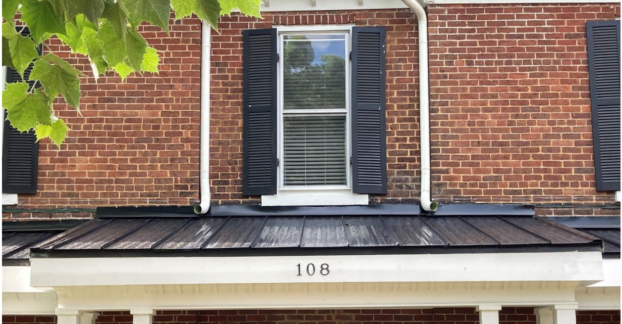
Replacement roof cladding with striations and ribs
