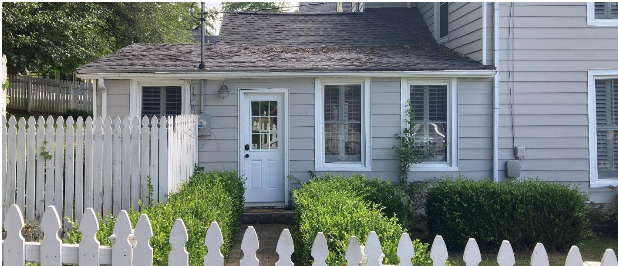
Southwest and West elevations of rear ell extending toward King Street
