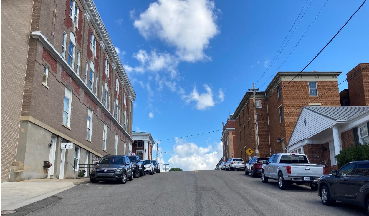
View of N. Court Street looking North
