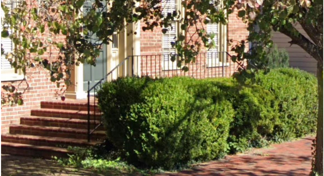
Previous wrought iron railing
