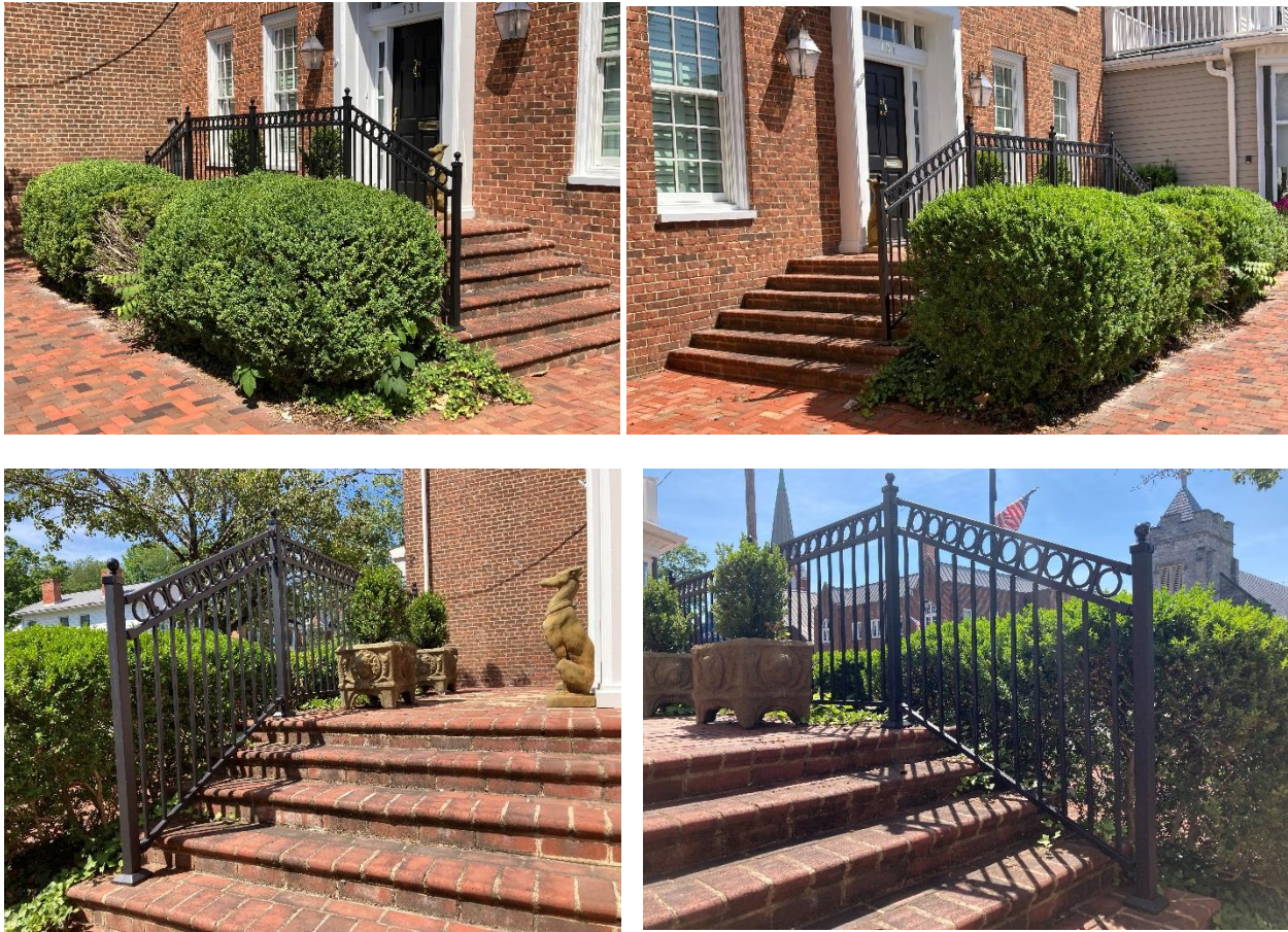
Unapproved cast iron prefinished black railing
