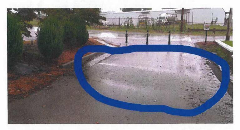
This water should be going down the gutter along Preston St. instead of down Hagy St. flooding the two houses and flowing across Country Boy Seed and the auto repair shop.
