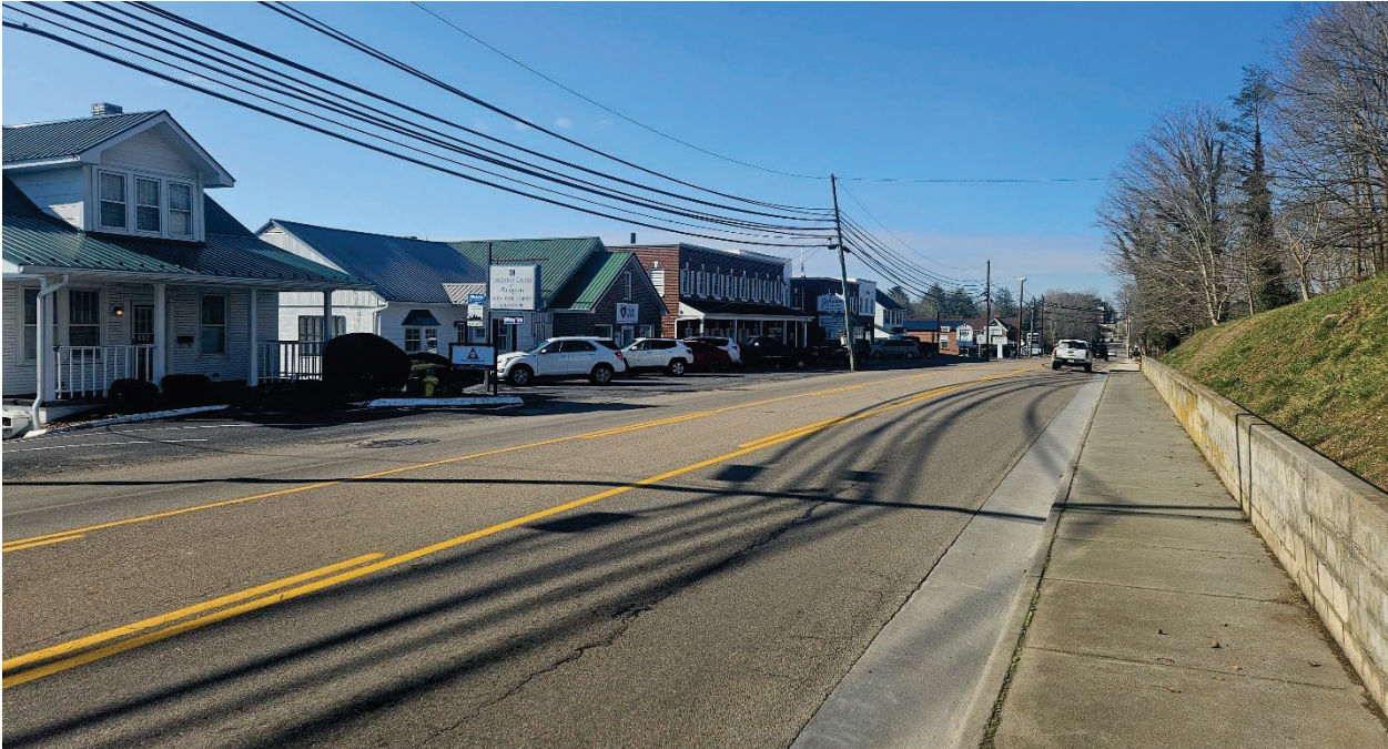
Street view of 480 W. Main Street looking West
