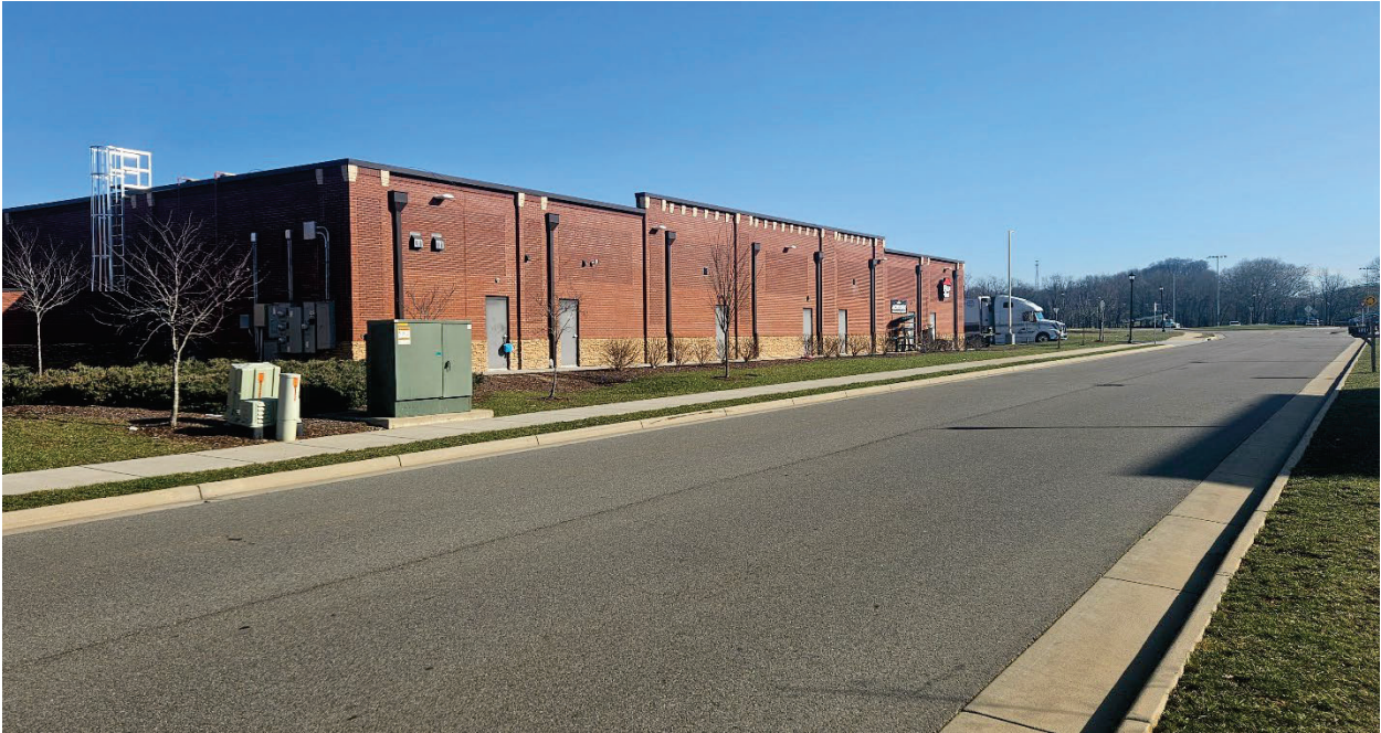
Street view of 117 Cook Street looking East
