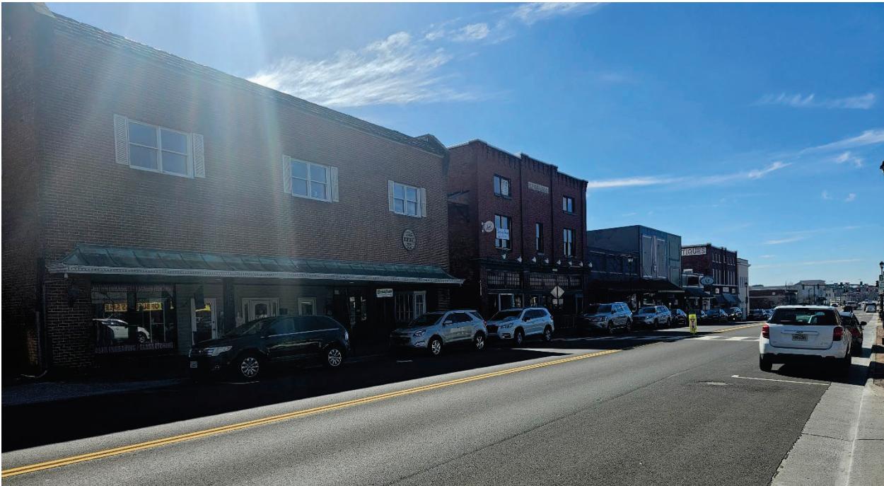
Street view of 252 W. Main Street looking West
