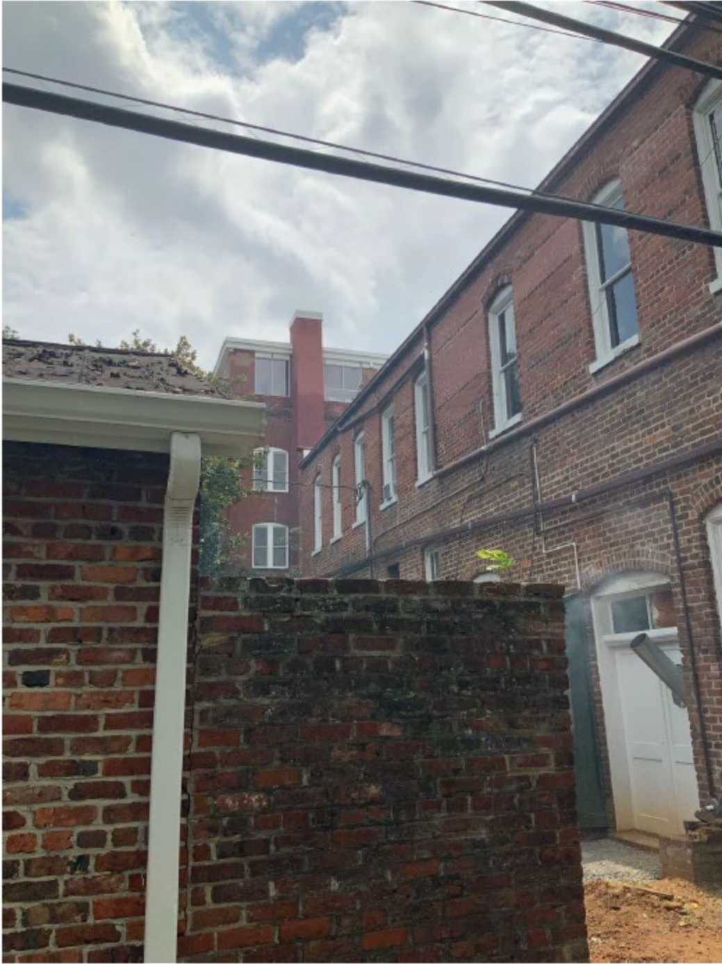
View from Plumb Alley
