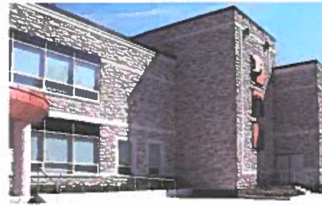
Abingdon Multi-Use Complex, Abingdon, Virginia | Architect: HOK | Product: Citadel® | Color: Custom
