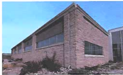
Abingdon Multi-Use Complex, Abingdon, Virginia | Architect: HOK | Product: Citadel® | Color: Custom
