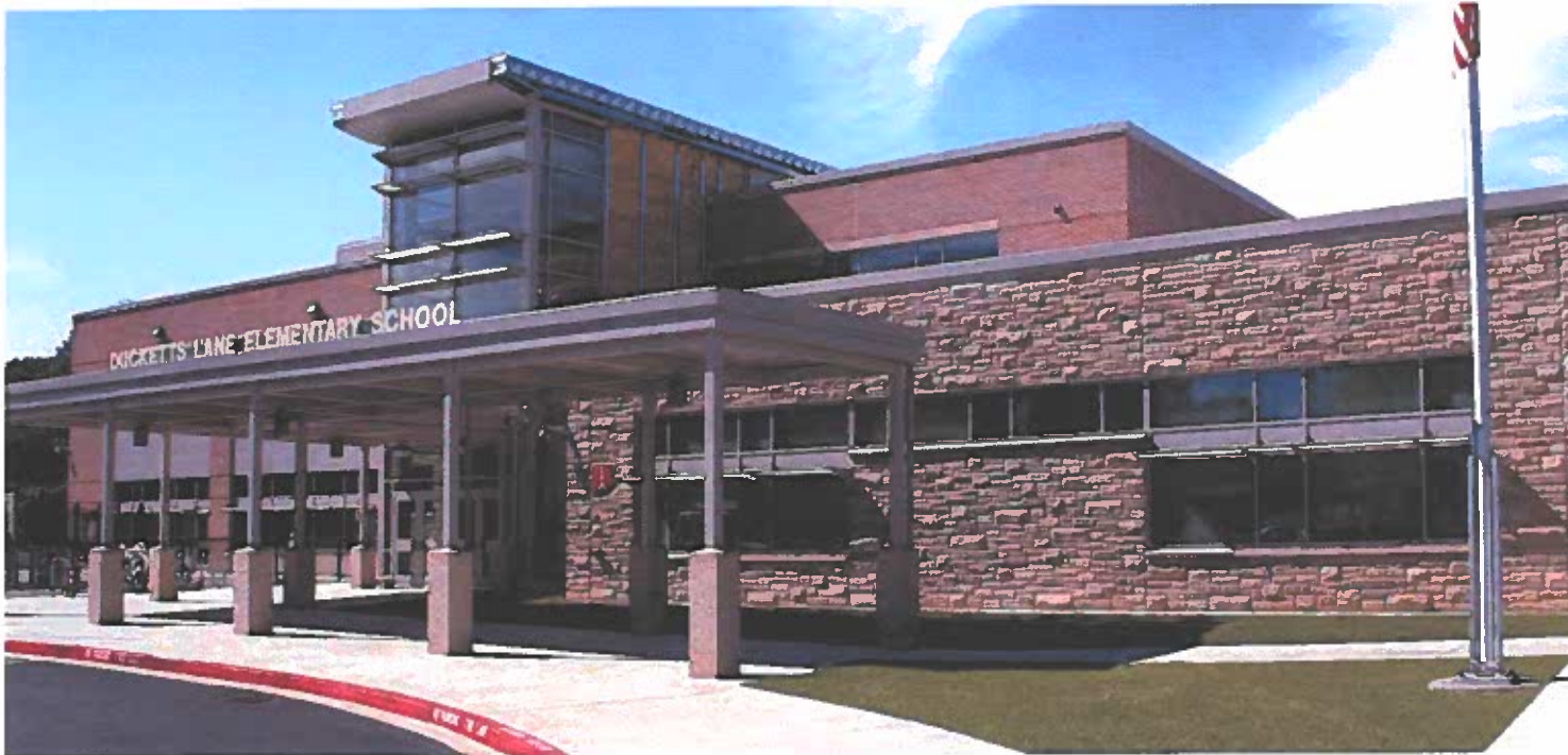
Dicketts Lane Elementary School, Abingdon, Virginia | Architect: HOK | Product: Citadel® | Color: Custom
